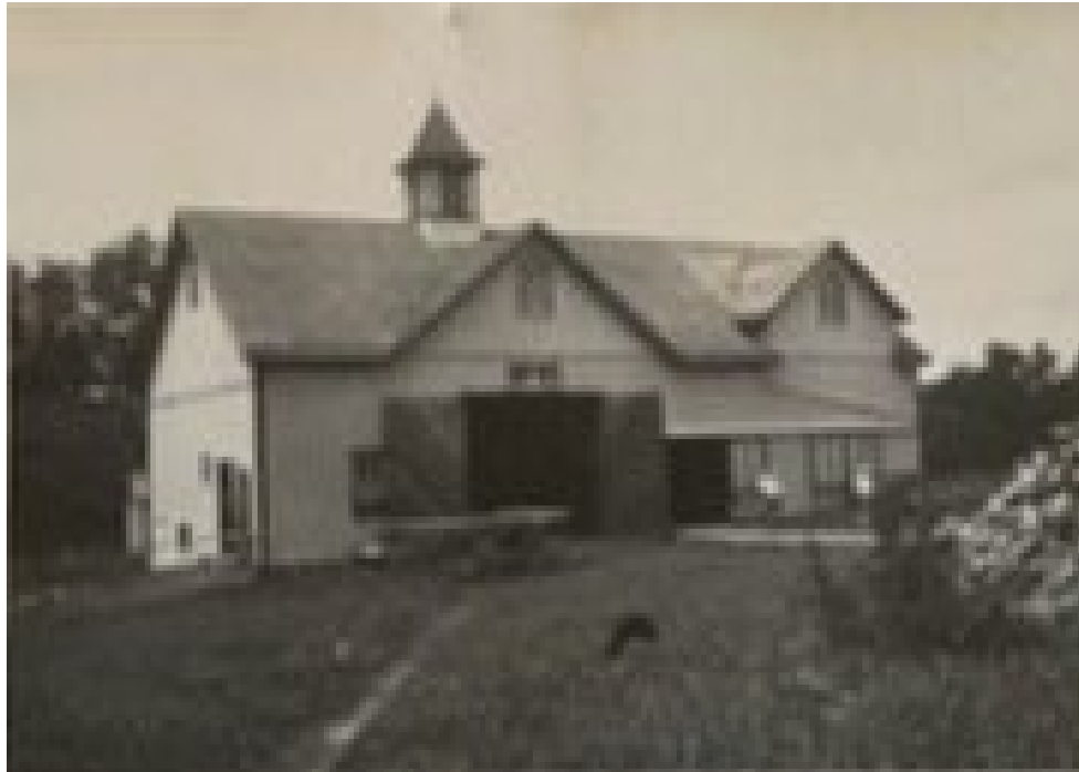
Figure 2.16 Circa 1900 photograph of the barn built by Joseph Wakeman Mather and William F. Mather. This original barn was located 120 feet west of the Main House. Courtesy MHF.
