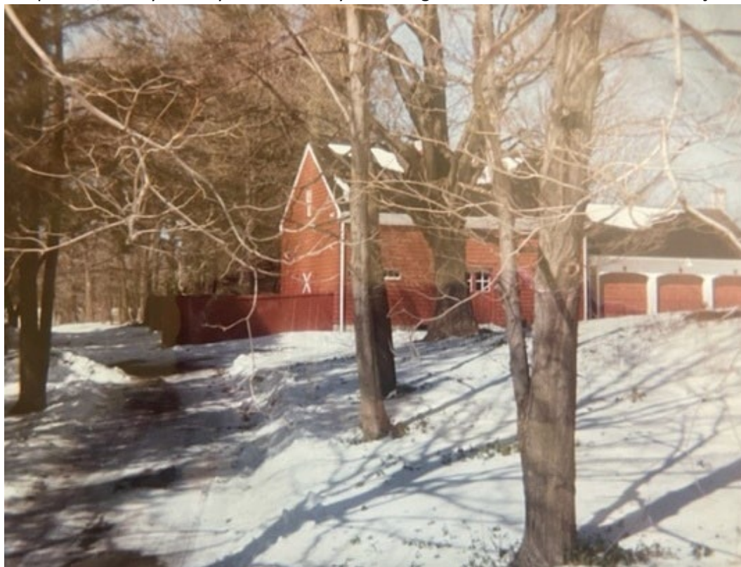
Figure 2.65 1982 photograph of a snow-covered view along the entry drive from Stephen Mather Road, lined by deciduous trees on either side. The Stephen T. Mather barn appears on the right. Courtesy MHF.
