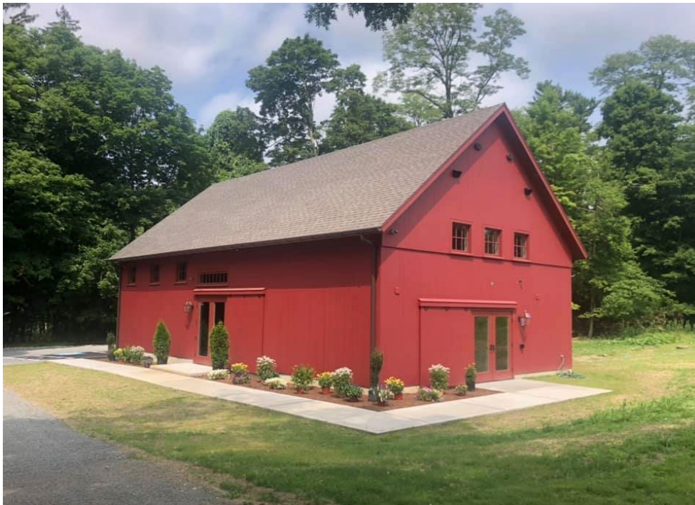
Figure 3.6b The Elizabeth W. Chilton Education Center, or the Barn, was built in 2020. A concrete walk wraps around the south and east sides of the building, providing access to two entries. Note the beds, not yet planted, between the walk and the facades. A wide strip of turf lawn divides the walk from the gravel drive. Courtesy MHF.
