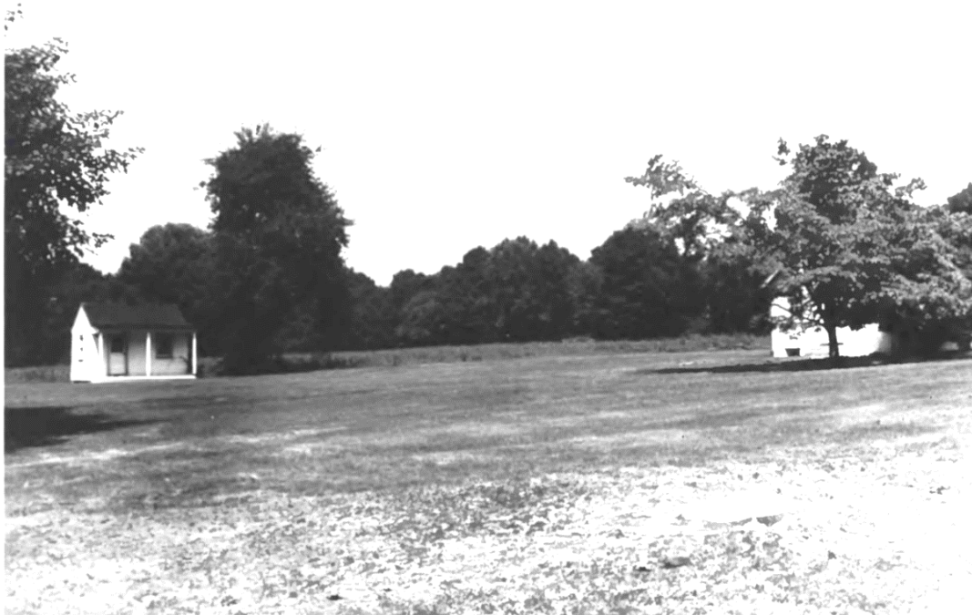
Figure 4.15a Circa 1963 photograph of the playhouse (left) and greenhouse (right). An open expanse of rough and patchy turf covers the foreground. Taller grass is seen in the background, to the north. Two trees are present, one near each of the respective structures. Courtesy MHF.
