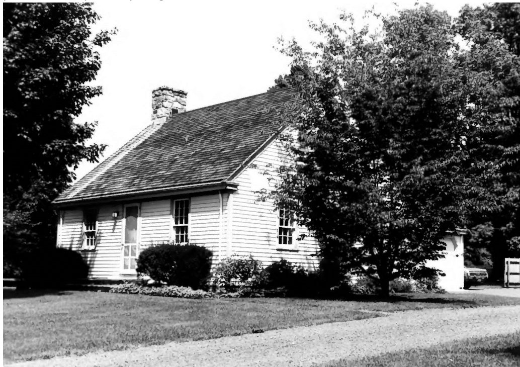
Figure 2.59 1974 NPS photograph of the Little House, added by Bertha Mather McPherson and built on the foundation of the former caretaker's cottage, located north of the Main House. Shrubs and groundcover beds line the cottage foundation. A narrow path leads from the gravel driveway to the front entry. Courtesy MHF.
