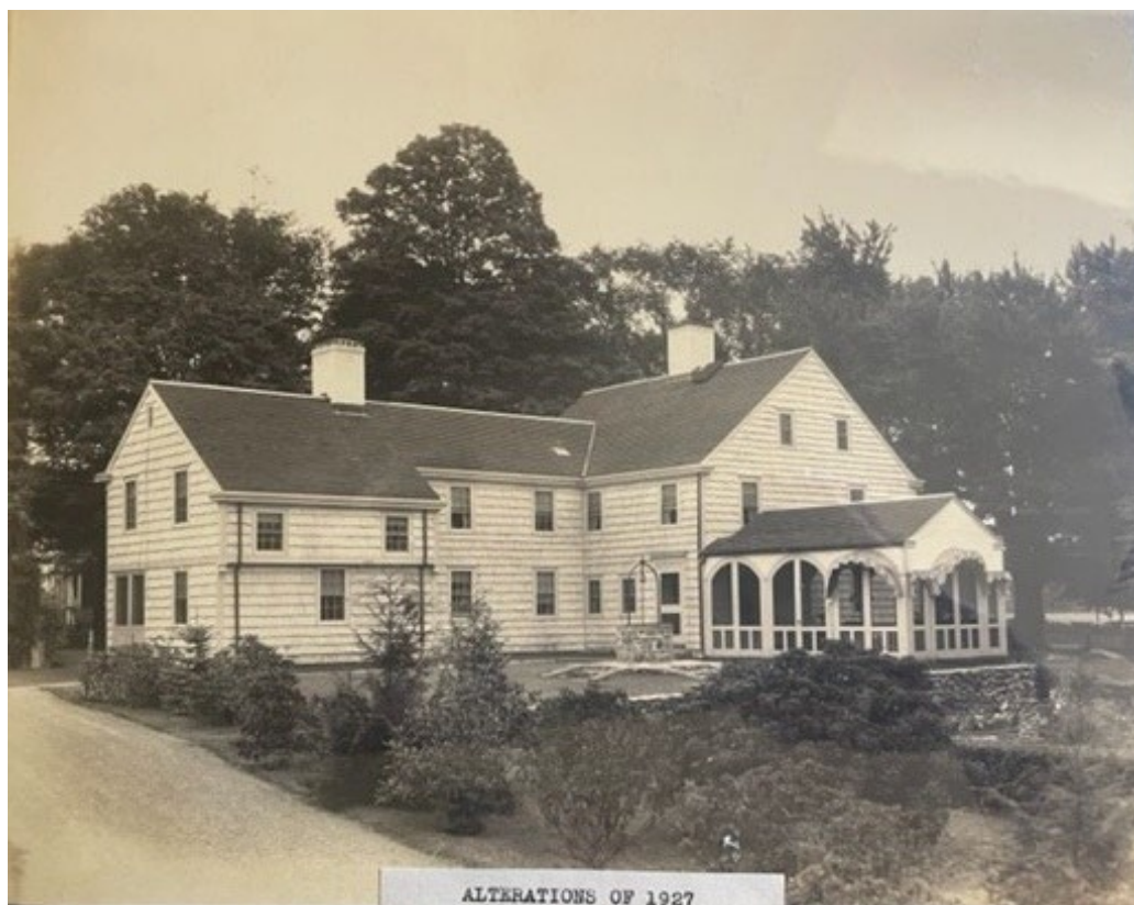
Figure 2.34 This ca. 1927-35 photograph of the house captures the new stone-and-iron wellhead, having replaced the 18 th -century wooden wellhouse. The 1927 alterations completed by Stephen Tying Mather and architect Thomas Harlan Ellett are shown, including a two-story addition (left) and a redesigned side porch. A bed of small evergreen trees and shrubs lines the gravel driveway. Courtesy MHF.
