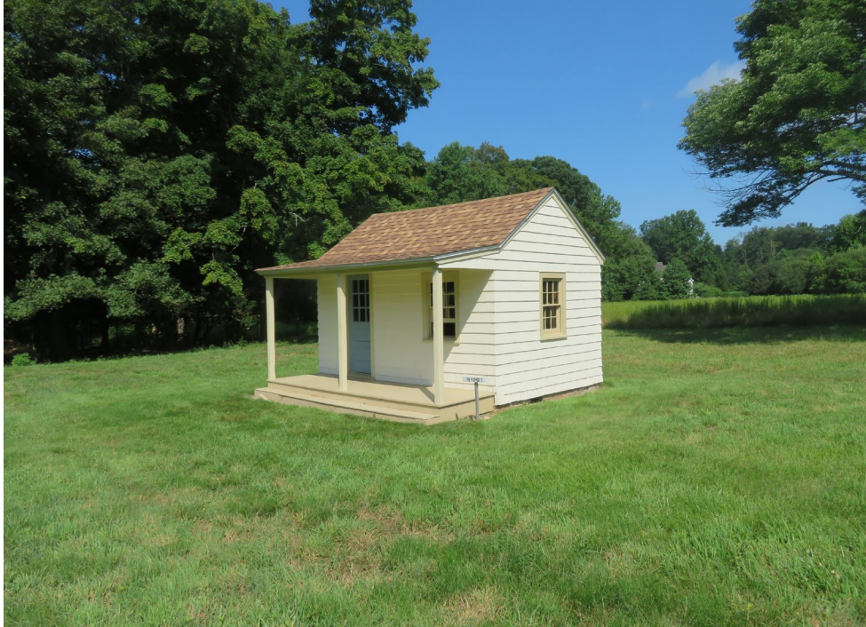
Figure 3.25 The playhouse is situated in the mown turf lawn, formerly marking the southern end of a small orchard of fruiting trees as seen in the 1934 aerial. This simple wood structure is set on a concrete footing and has a small wood porch, two steps above finish grade. The playhouse was recently restored in (0000) and is open for use by visiting children today. HL 2023.
