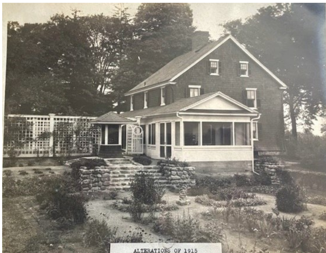
Figure 2.30 Circa 1915 photograph of the west side of the house shows the newly constructed one-story screened porch and the as-constructed Walter Burley Griffin garden with geometric beds. Courtesy MHF.
