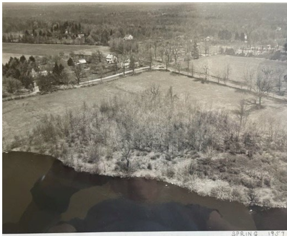
Figure 2.46 1954 oblique aerial photograph of the Mather Homestead in context. Mathers Pond is seen to the southwest, at the bottom of the image. Stephen Mather Road extends east from the left side of the image, and Brookside Road extends north from the right side. The Homestead is situated on the north side of Stephen Mather Road. Courtesy MHF.
