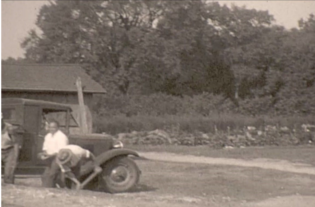
Figure 4.18a This circa 1929 still image capture shows the northwest view from the same vantage as the previous figure. A service drive divides the vicinity of the barn from the cultivated vegetable beds and row crops to the north (right). The same outbuilding seen in the previous figure appears at the left side of the image. Further west, beyond the cultivated area, a dense shrub edge and mature deciduous trees are present. Courtesy McPherson-Nickerson family.
