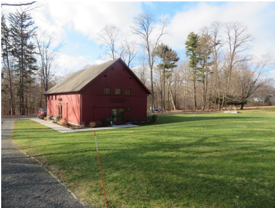
Figure 4.19b In 2024, the Education Center is present in the approximate location of the 1929 barn. The gravel drive does not extend up to the foundation of the structure; a concrete walk wraps around the perimeter, providing access to the east façade entry. The maple trees north of the historic barn are not present. Mown lawn extends north alongside a wooded area to the northwest. HL 2024.
