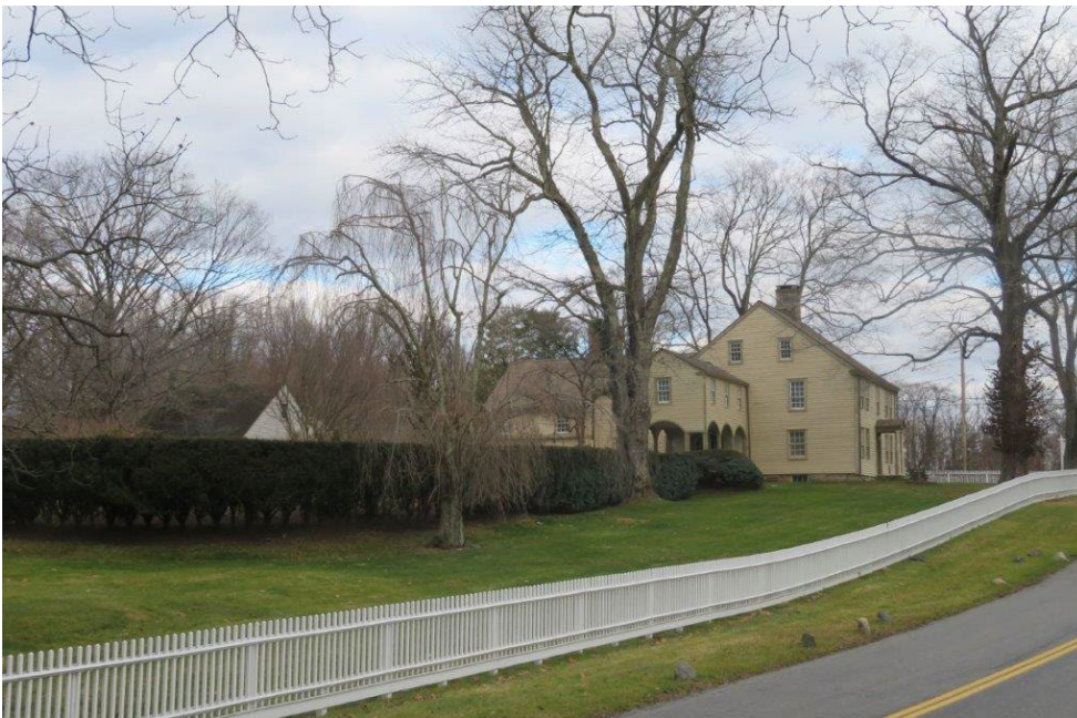
Figure 4.2b Repeat view in 2024 shows the same gentle grade rising to the west along Stephen Mather Road toward the Main House. The Little House, built in 1965, is one story shorter than the former caretaker's cottage, and the increased height of the yew hedge around the Sunken Garden partly obscures the view of the smaller structure. Mature shade and flowering trees stand between the Sunken Garden and the road, which is lined sporadically with stones to discourage parking. HL 2024.
